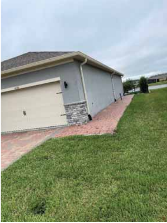
3692 Beautyberry Way: Fence constructed within easement.
